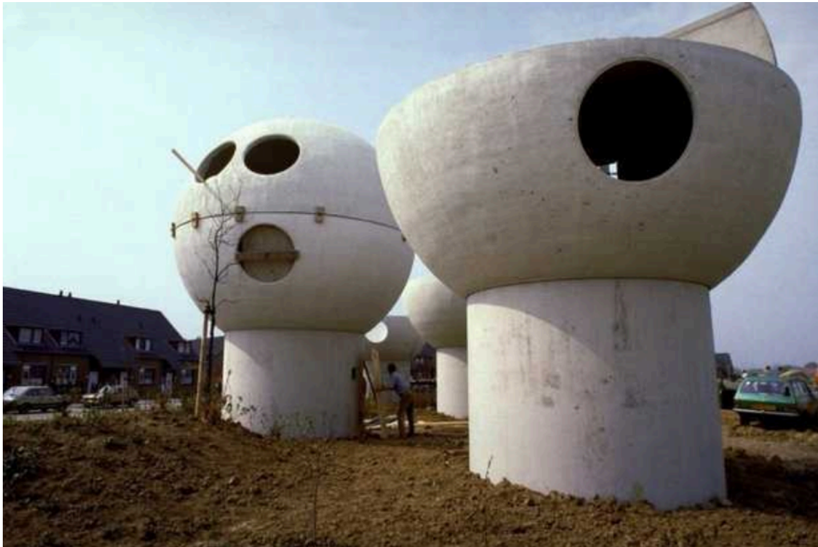
Figure 14 “Bolwoningen” under construction. The sphere is made from fiberglass instead of traditional materials like concrete (Merin).
